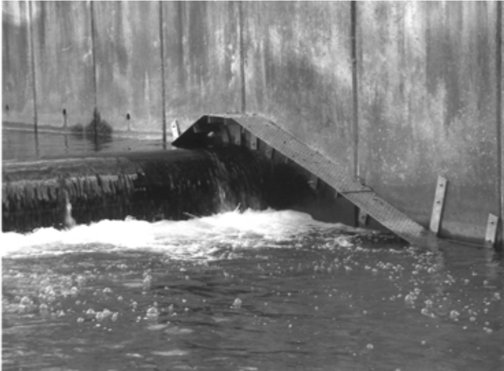
Figure 3 - Otter ramp over a weir where five casualties had occurred prior to its installation
